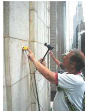
Testing for internal cracking and debonding of terracotta cladding
