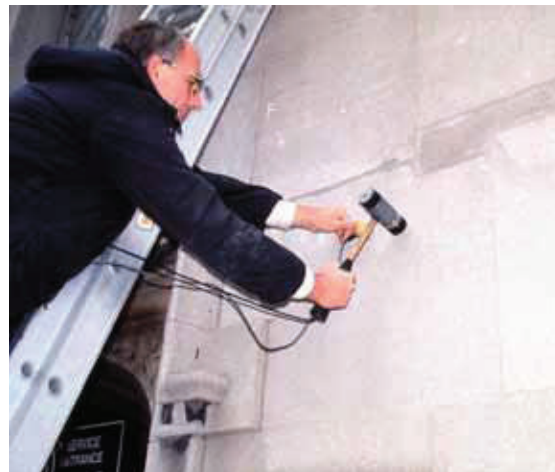
Testing for cracking and debonding of limestone cladding
