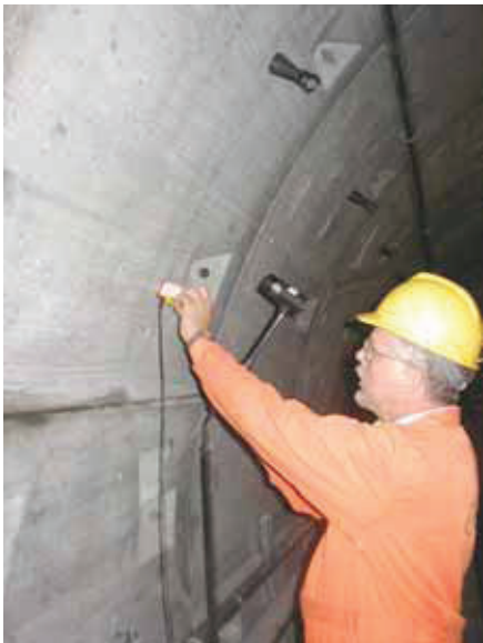
Testing for voids behind tunnel lining
