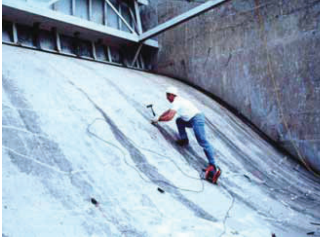
Testing for delaminations in dam spillway
