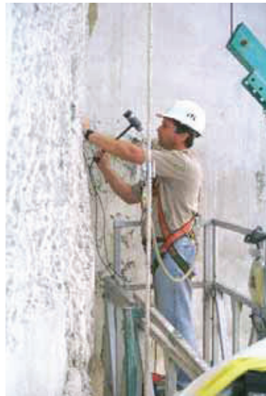
Testing for honeycombing in slip-formed silo
