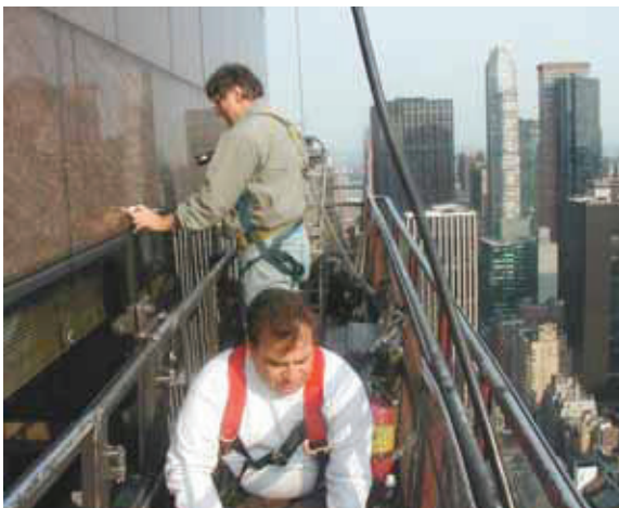
Testing for anchoring quality of granite panels in high-rise building
