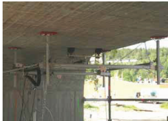
Vacuum scanner attached to soffit of post-tensioned bridge
