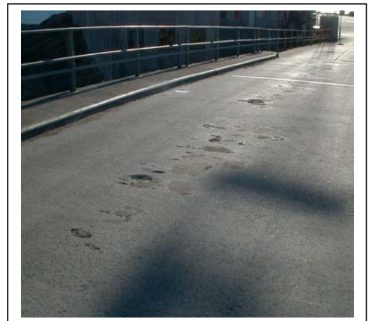
Fig.11. The first picture shows the corroded reinforcement and some water from cooling the diamond cutting blade. The second picture shows the damage and the mortar repairs.
