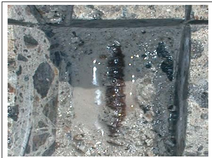
Fig.11. The first picture shows the corroded reinforcement and some water from cooling the diamond cutting blade. The second picture shows the damage and the mortar repairs.
