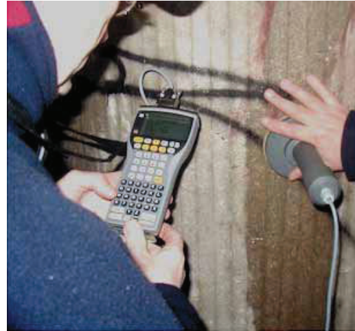
Highway bridge column being tested for corrosion rate with the GalvaPulse
