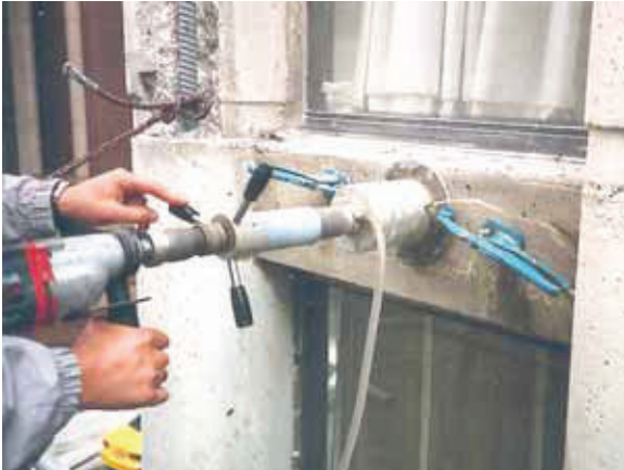
Coring with the CS-75 rig clamped to the surface
