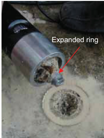
View of valid CAPO-TEST of a slab. Note the well formed failure ring on the surface of the slab.
