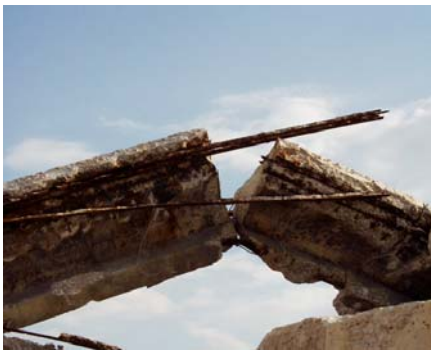
Figure 3. Span structure (T-beams)
