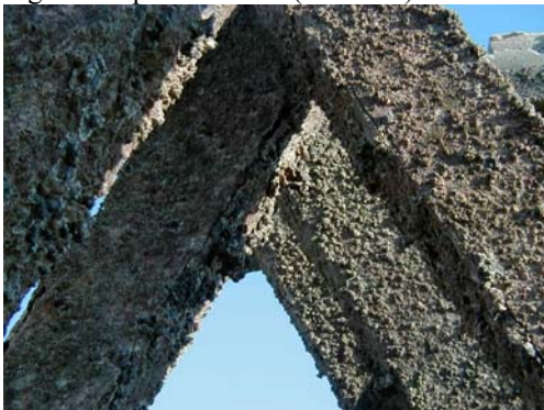
Figure 5. Columns of the tested deck covered with shells
